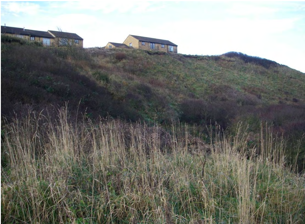
Plate 12. Site view of Behaviour Unit II showing over steepened back-scarp below Upper Plateau.
