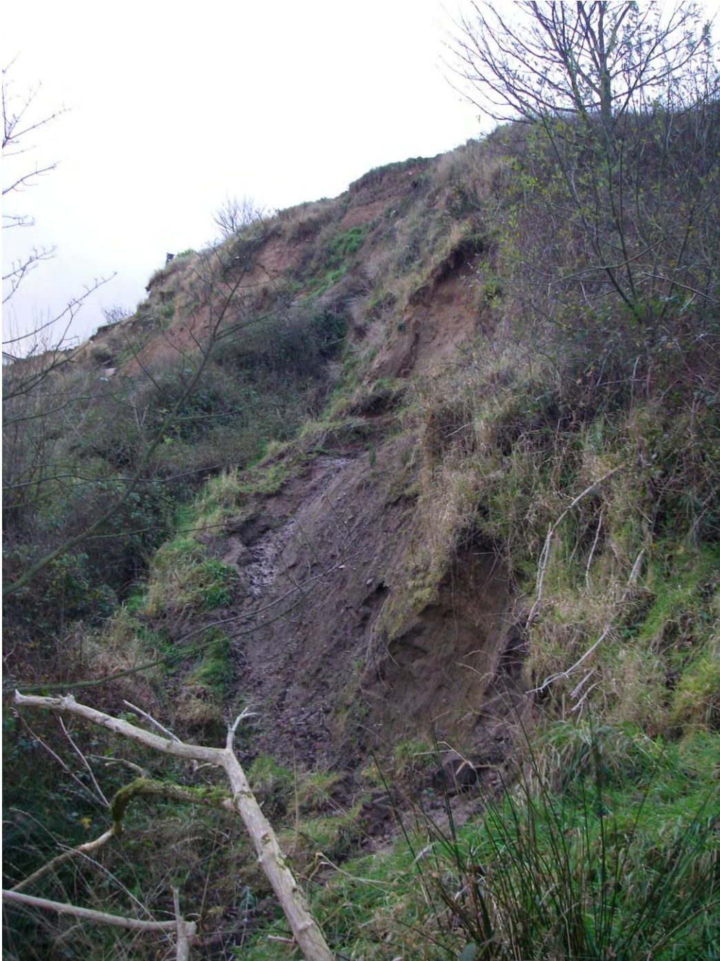
Plate 39. Site view (taken below Plate 33) of backscarp showing groundwater issues.
