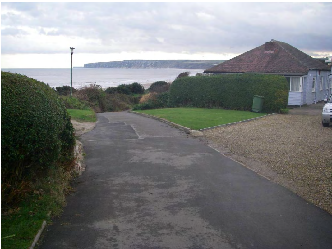
Plate 58. Site view looking down slope from 'level' mid-slope bench.
