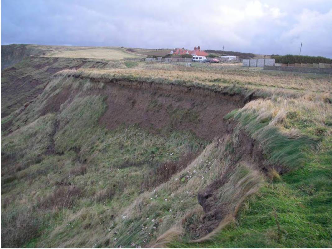
Plate 40. Site view looking south across Killerby Cliffs.
