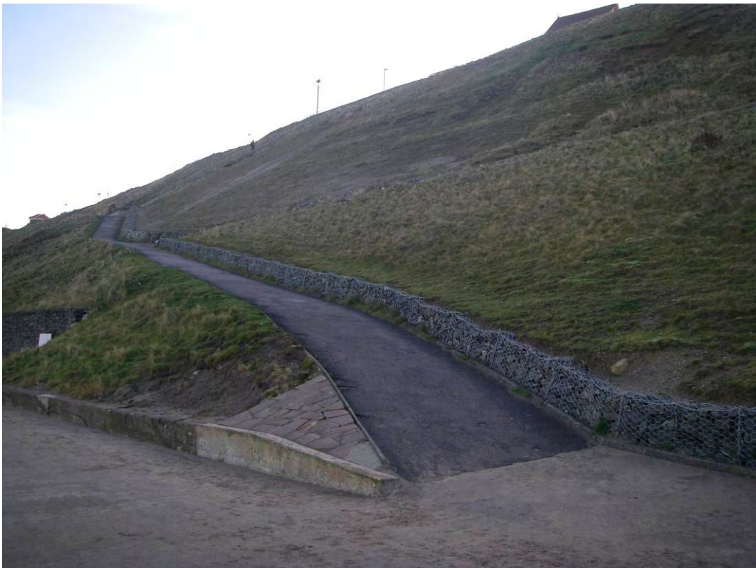
Plate 8. Site view of West Cliff slopes looking east.
