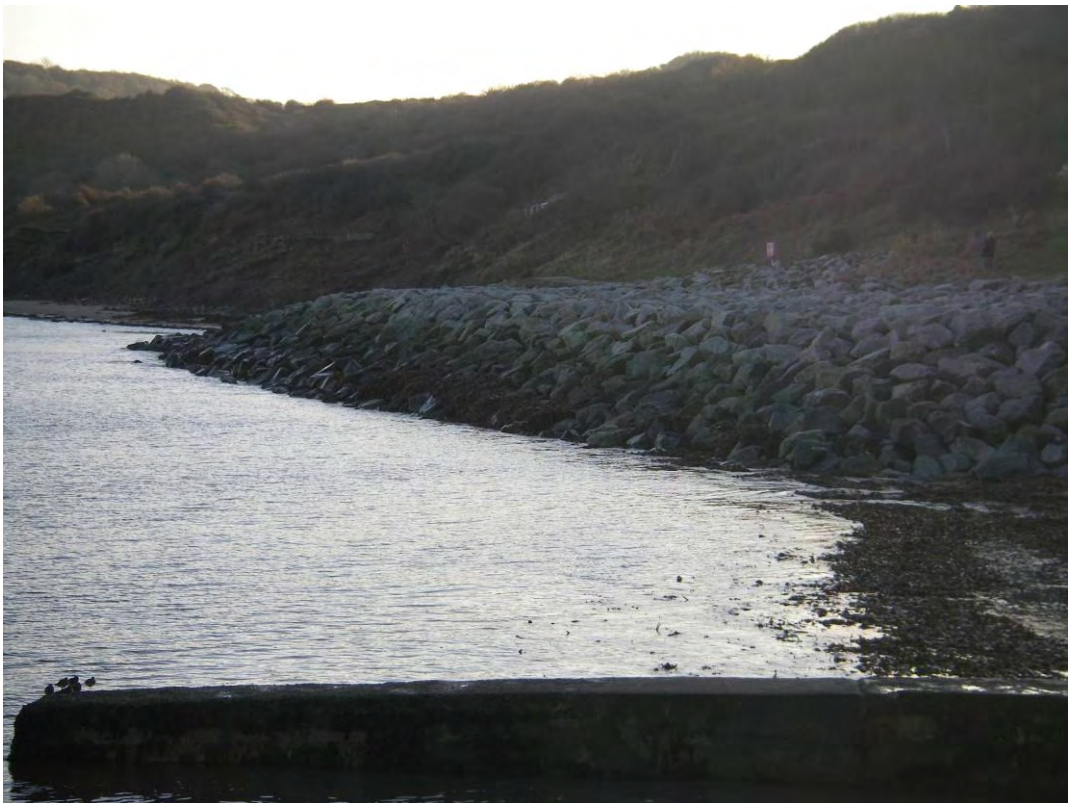
Plate 4. Site view looking south-south east across rock armour revetment towards Dother Pits.
