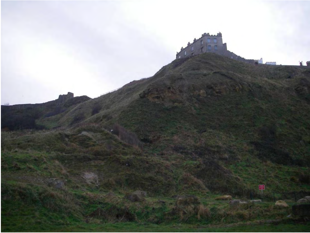
Plate 17. Site view of The Holms looking up towards Castle by The Sea.
