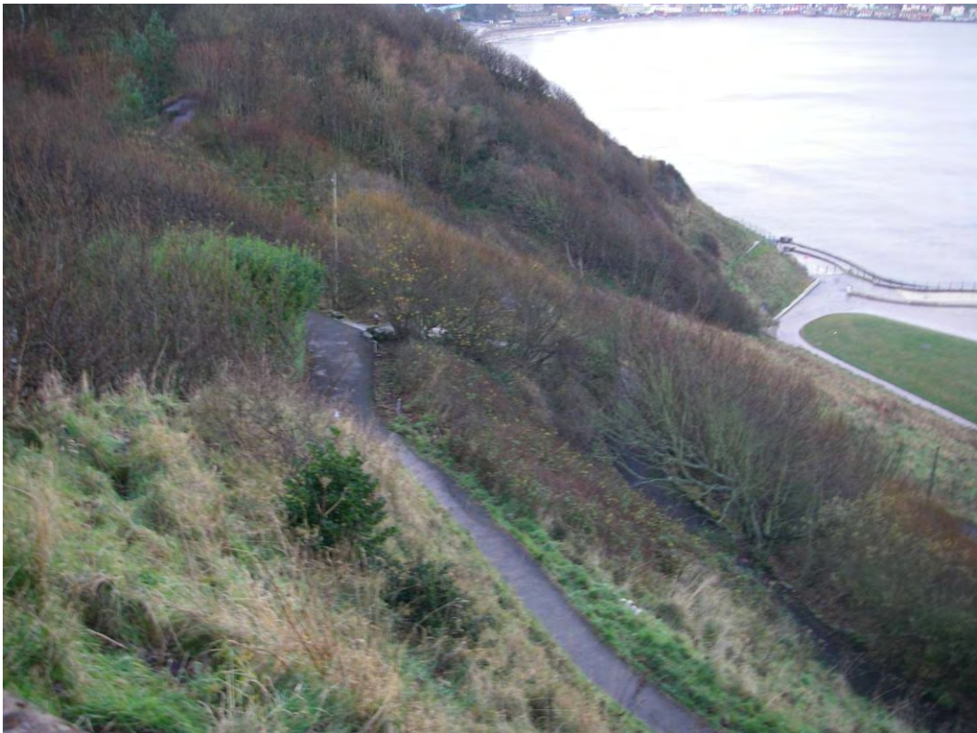
Plate 22. Site view of steep slope angles above South Bay Pool Cliff.
