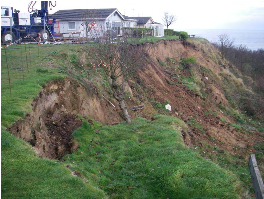
Plate 35. Site view looking north east along regressing crest showing recent failure.
