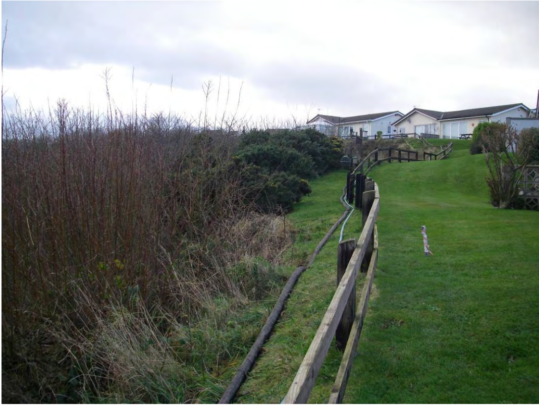
Plate 31. Site view looking south west along crest of Cayton Cliff.
